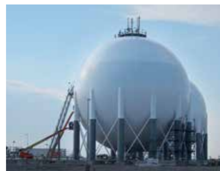
Spheres including legs and bracing
