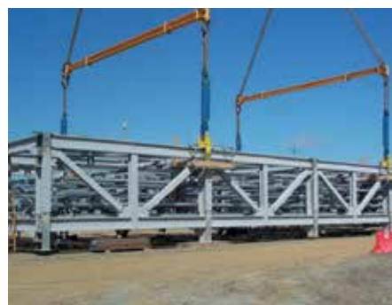
Modular steel structures
