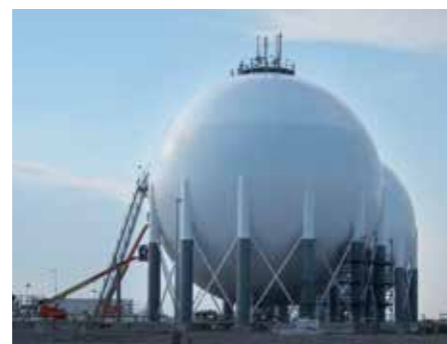
Spheres including legs and bracing
