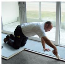
The boards are mechanically fixed by means of staples or screws. The screws must not exceed the thickness of the supporting structure or blocks in order not to create a structural path for noise transmission.
