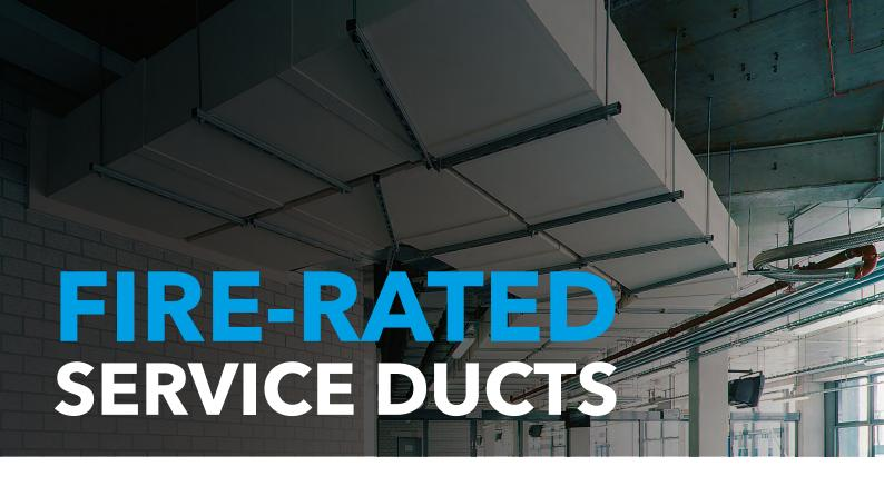
Fire-rated service ducts are specially designed to withstand high temperatures and prevent the spread of fire and smoke through building services such as electrical cabling, and plumbing. They are tested and certified to maintain their structural integrity, insulation, and cable functionality for a specified period—typically 30, 60, 90, or 120 minutes.
