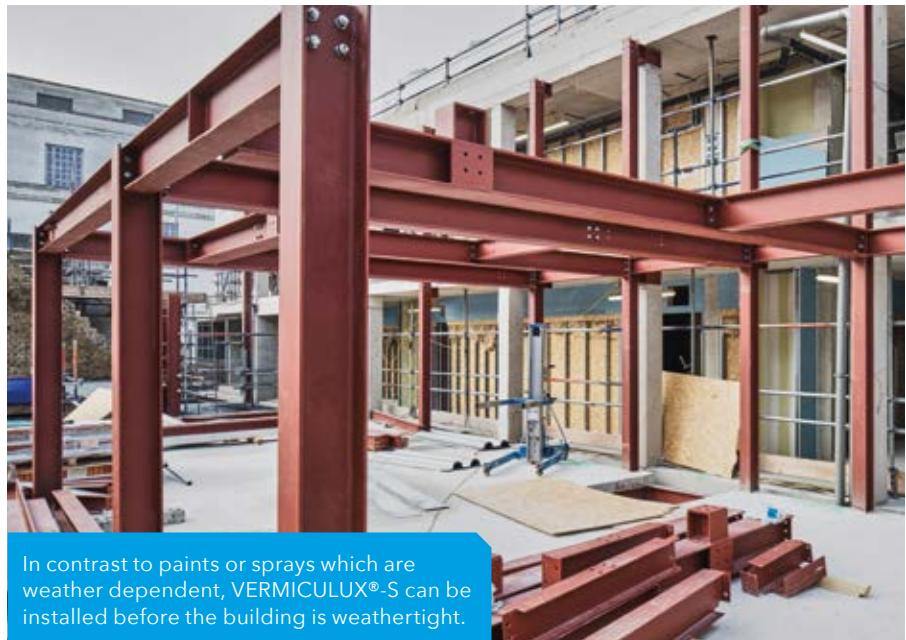
In contrast to paints or sprays which are weather dependent, VERMICULUX®-S can be installed before the building is weathertight.
